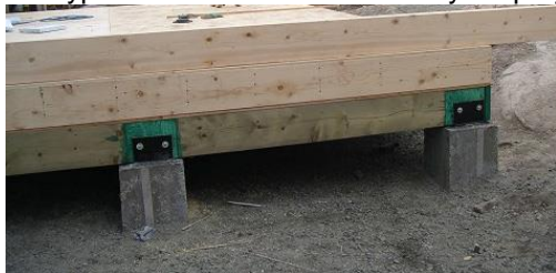
Figure 5: An example of a concrete pile foundation
